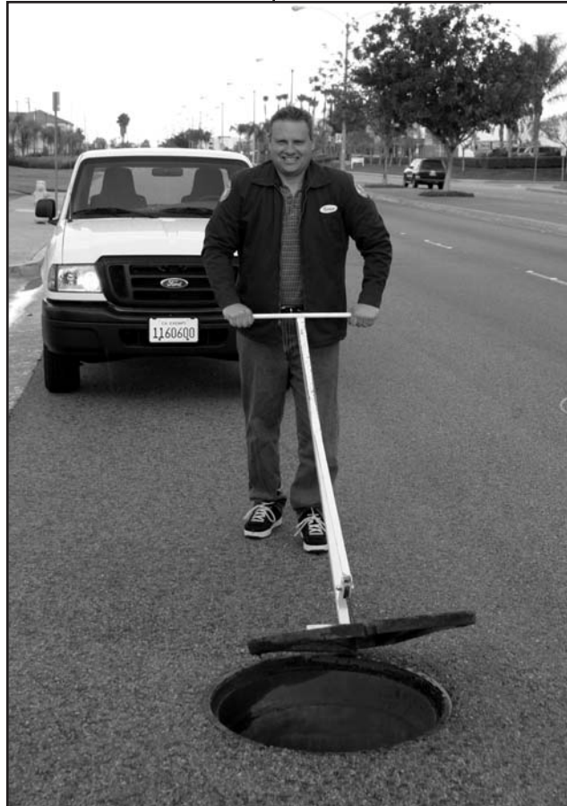
Underground Storm Drain Foreman Kevin Vargas lifting a manhole cover
